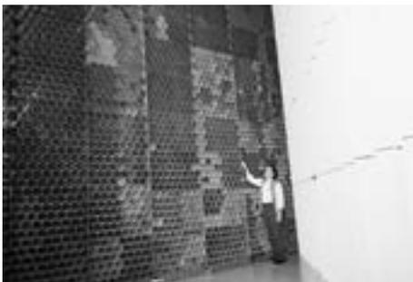
*This honeycomb installation is from a Boeing transonic wind tunnel in the 1960s.*
